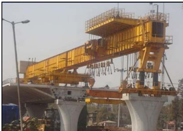
F-5.11 Segment being lifted and placed
