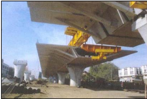
F-5.13 Segment being placed in position
