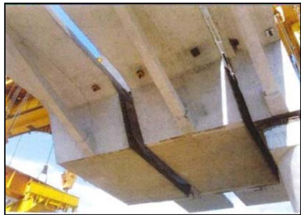
F-5.12 Placing of segment in order
