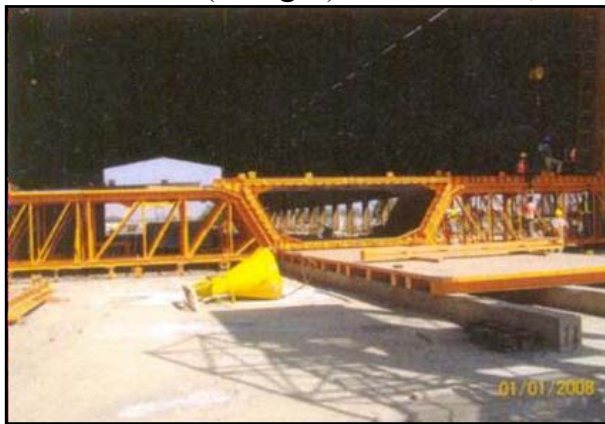
F-5.9 Formwork of the Segment at the casting yard
